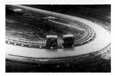
3. In 1973, in a beet field near the Orly Airport runways, the first cars of the first Aramis prototype were tested. This photo shows the test track, along with two little cars that are running quite close to each other, even though they are not mechanically coupled. [Photo RATP]
