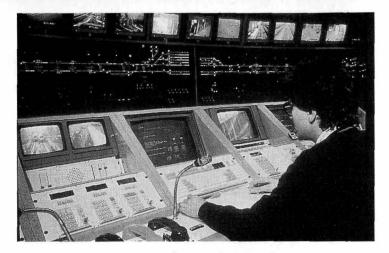
7. The control room for VAL in Lille. The success of big brother VAL cast a shadow on little Aramis. A major innovation: the former drivers are now positioned in front of a control panel, and regulate the movements of the automated trains from a distance. [Photo Matra]
