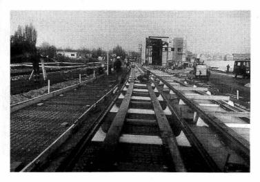
10. The construction of the experimental site is well under way. This photo was taken from the eastern side of the workshop. Beside the tracks the guide rails and electric power supply rails are clearly visible, along with the guides for the rubber tires. [Photo RATP]
