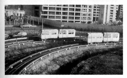
13. After the two pairs of cars have passed a branching point, each pair goes its own way, thereby feeding—without transfers—the transportation networks that a traditional line would be unable to serve. [Photo RATP]
