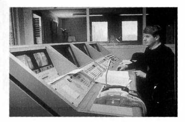
14. Aramis' Central Command Post. As with VAL (whose control room is shown in Photo 7), the wholly automated system is not intended to have any human actors except at the two extremes: the passengers riding in the cars, and the controller at his desk. [Photo Matra]
